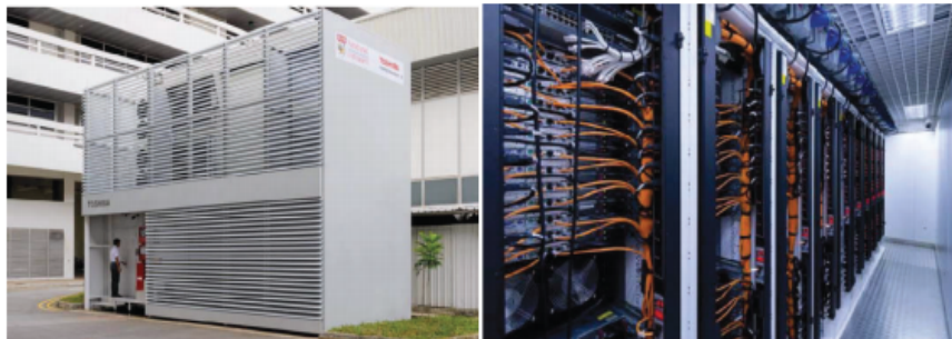
Fig. (3). A Modular data center was built at Nanyang Technological University (NTU) for System/Tested Research. The tested hosts 270 servers organized into 10 racks.
