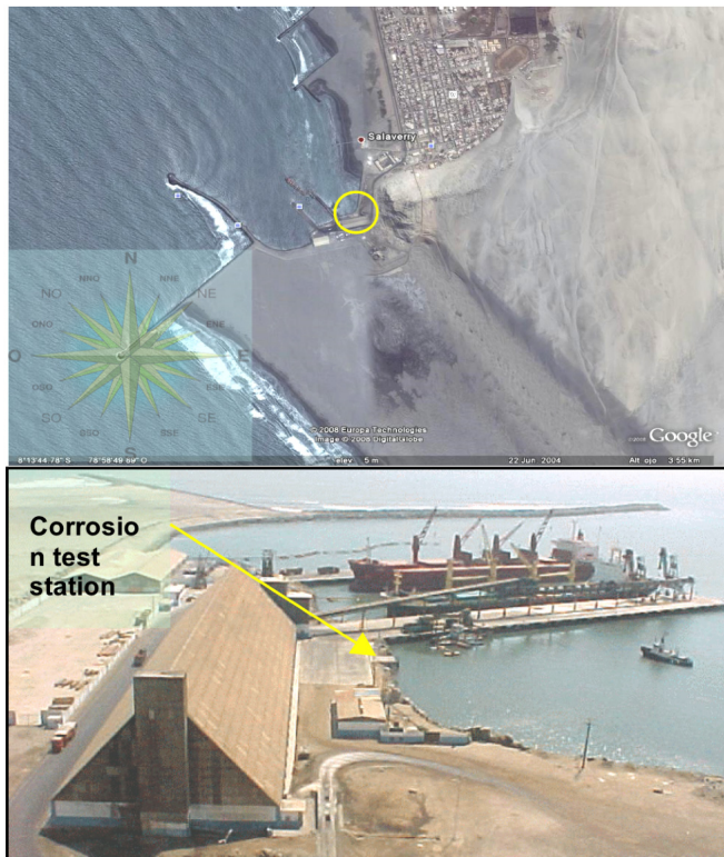
Fig. (2). Aerial photographs of Terminal Portuario Salaverry ( 8^{\circ}13'40,57'' S; 78^{\circ}58'54,60'' W), showing (in yellow circle and arrow) the location of the corrosion test station and the environment that surrounds it: the areas of ships and crafts are zones of continuous dredged of silts.
