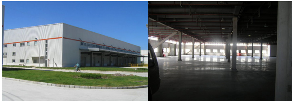
Fig. (4). Facility photos of site A.
