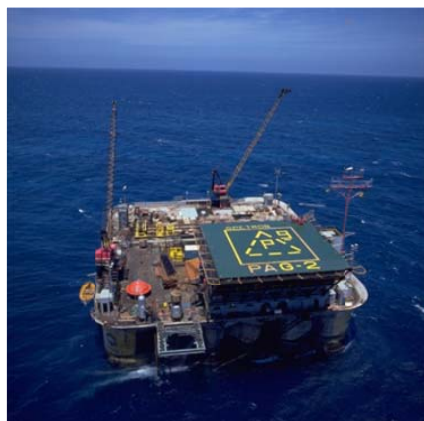
Fig. (9). Petrobras fixed platform located in shallow water (22 m deep) in the NE region of Brazil.
