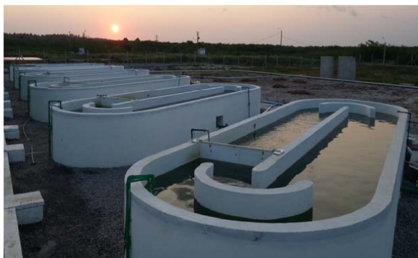
Fig. (7). Open ponds in the pilot plant running to produce microalgae for advanced fuels (author's personal archive).
