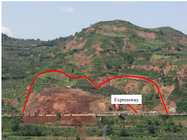
Fig. (2). Overview of the large landslide.
