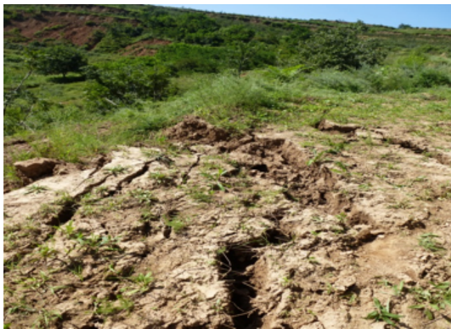
Fig. (3). Cracks at the trailing edge of landslide.
