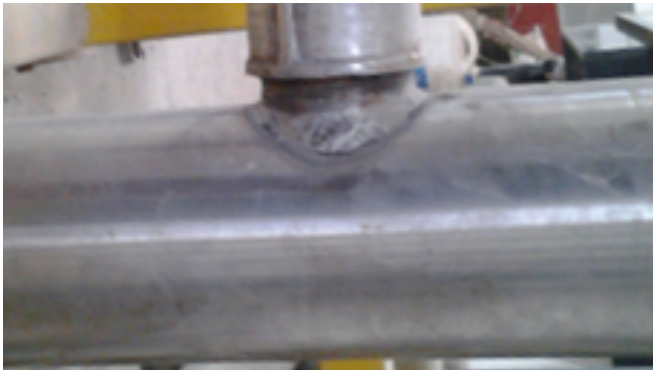
Fig. (8). Hydraulic test of tee.
