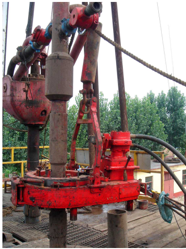
Fig. (17). Rotating liner by casing tong.
